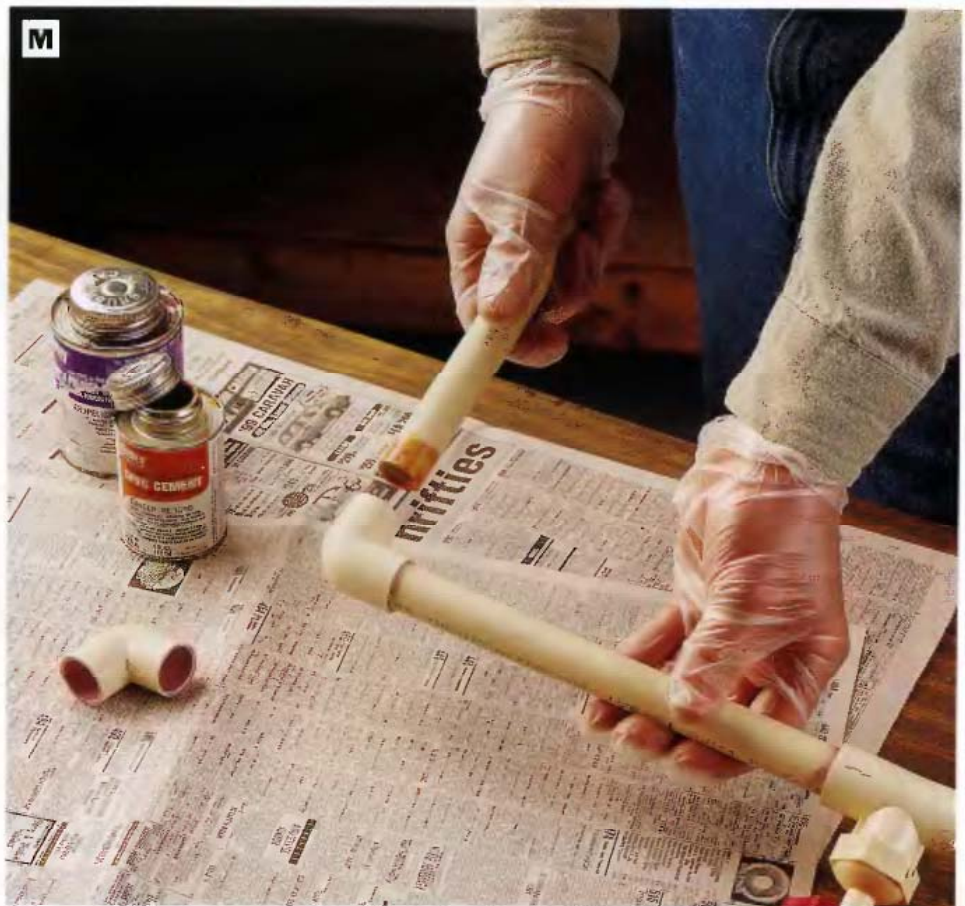
PHOTO M: Cut the straight pipe sections to length and dry-assemble the entire plumbing unit to check its fit on the potting bench. Then disassemble the PVC, prime the mating parts of each joint, and bond the PVC together with CPVC cement. Wear gloves when bonding the parts.
